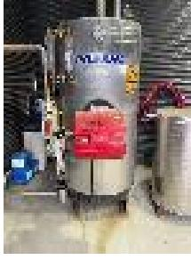
CONSOLIDATED FIRE & STEAM STEAM BOILER, MOD: PRESHA UT300, DOM: 2008, SERIAL: CFS0128, NAT GAS, 750KPA, 415V                                                                                                                                                                                                                                                 |      |
